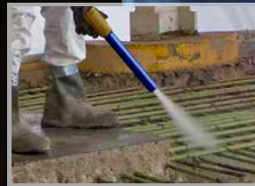
Concrete Repair and Restoration
