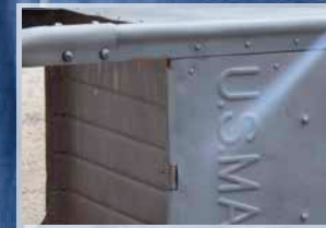
Steel Surface Preparation
