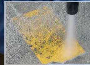
Concrete Cleaning and Surface Preparation
